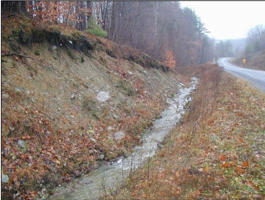
Typical Drainage Ditch, Excavated in Glacial Till, Lent Hill Rd.
